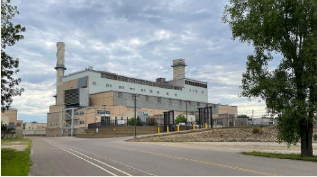
Black Dog Generating Station (Natural Gas)
