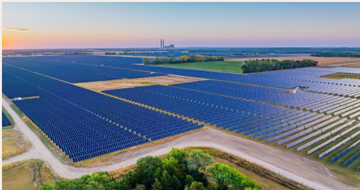
SherCo Generating Station (Solar & Coal)
